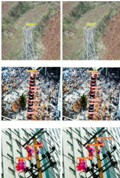
Figure 9. Fault Identification in a Typical Transmission and Distribution Inspection Scenario
