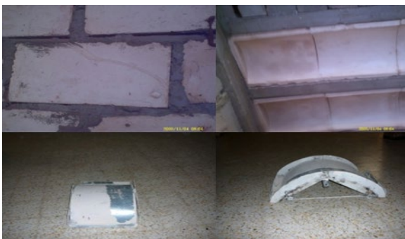
Figure 1. The use of gypsum blocks for the ceiling and walls in the city of Ouargla.
